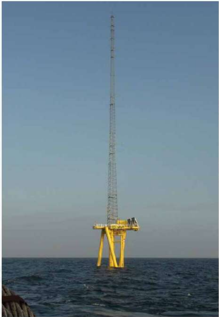
Figure 14 – Completed met mast with jacketed foundation (October 2010).
