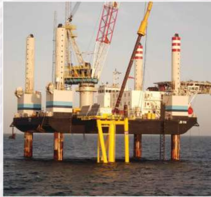
Figure 10 – Met mast installation (September 2010)
